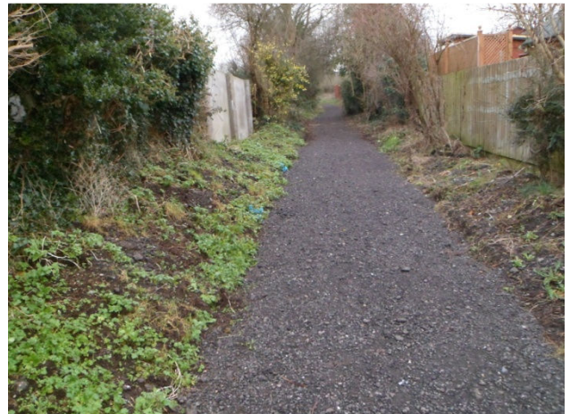
Byway 89 After Surfacing
